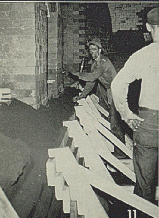
Fig. 10—Flat with exception of tap hole section has been rammed. Front and back banks are rammed at same time. Man in foreground is following hammer operator and shoveling loose Ramix behind form. When material has been tamped to within 1½ inches of top board, another plank is fastened to forms and procedure repeated
