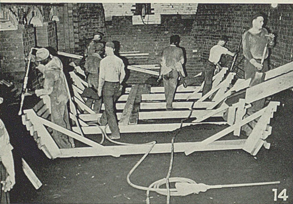
Fig. 12—Looking toward front of furnace showing completed Ramix sub-hearth. After forms are removed the junction of banks and flat is carefully rammed to insure good seal
