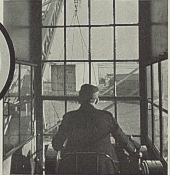
Interior view of crane-cab at eastern railroad pier, showing compact EC&M Master Switches conveniently grouped within easy reach of the operator.
