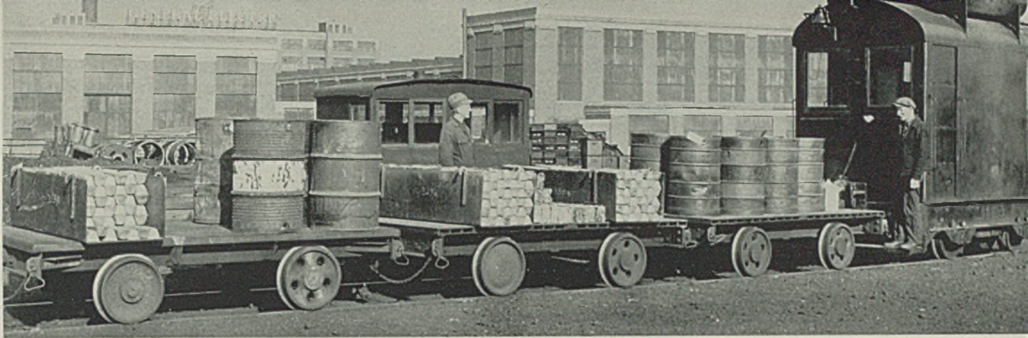
Fig. 1. (Left, above)—Trays are taken to salvage section on flat cars which are same size as tray—5 x 10 feet. Nonferrous metals are accumulated in drums and taken to salvage section as shown in Fig. 2
