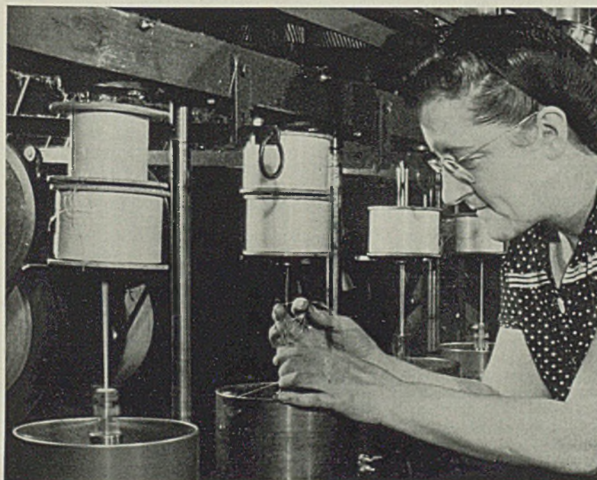
Fig. 2—Sun glass replaces asbestos in insulation for copper wire. Operator is inspecting the glass strands before they are machine-woven around the wire
