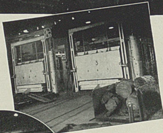
↑ Amsler-Morton Car Type Annealing Furnaces. Sidewalls insulated with SII-O-Cel C-22 Brick backed up with Superex Block. Roof of same materials plus 1" J-M No. 500 Cement.
