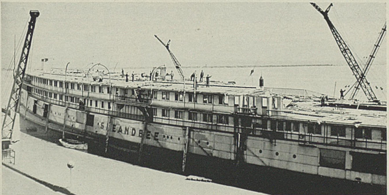
CLEVELAND: Largest passenger ship on the Great Lakes, the 500-foot SEEANDBEE is being overhauled and the upper decks reconstructed to carry airplanes for training Navy fliers. The vessel was built in 1913 for Cleveland-Buffalo service. NEA
