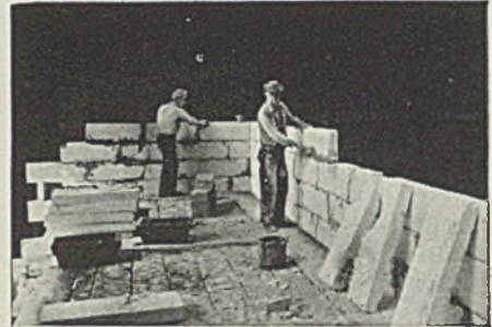
Suporex Blocks —The outstanding block insulation for temperatures to 1900° F. Combines high heat resistance with low thermal conductivity. Standard sizes 3" x 18", 6" x 36" and 12" x 36"; from 1" to 4" thick.
