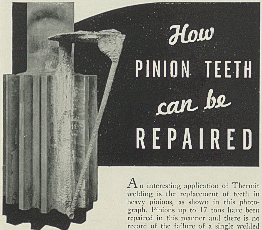
Pinion Repaired by Thermit Welding. Risers and Gates Not Yet Removed.
