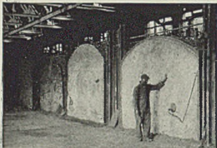
SII-O-Cel C-3 Concrete —Cast on the job from SII-O-Cel C-3 aggregate and cement. Sets up into a durable semi-refractory insulating concrete for use up to 1800° F. 28 lbs. required per cu. ft. Shipped in 100-lb. bags.
