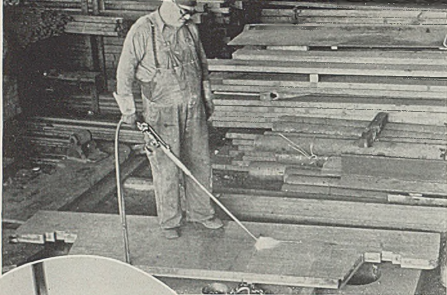
Upper left—Flame descaling steel plate before application of metal filler as a base for higher-luster finishes proved to be more economical and faster than sand-blasting. It can be accomplished either before or after shape-cutting and machining of the plate
