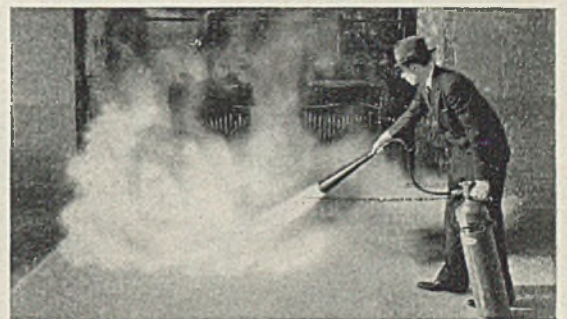
Extinguishing a transformer fire with C-O-TWO Portable Unit
