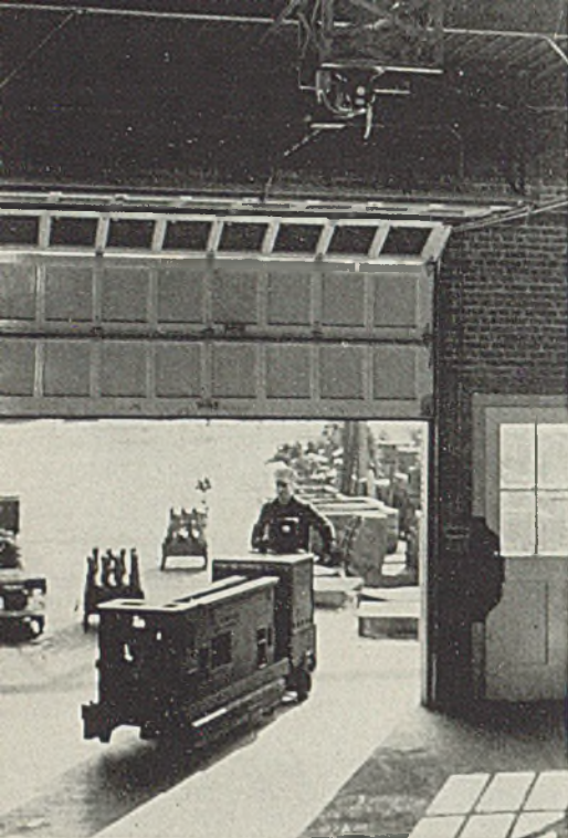
Fig. 4. (Left)—Door is raised automatically to permit truck to enter when driver presses control button on truck and drives over pickup coil in driveway
