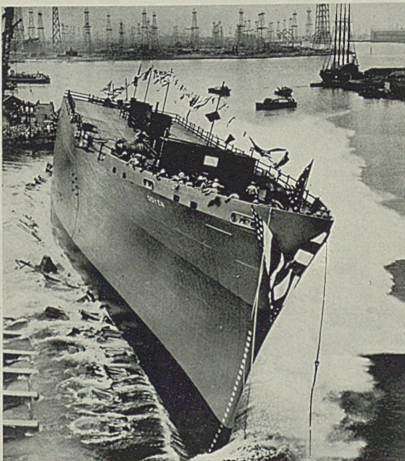
NAVY transport vessel, U. S. S. DOYEN, slides sidewise down the ways in recent launching at Consolidated Steel Corp.'s Long Beach, Calif., shipyard. NEA photo
