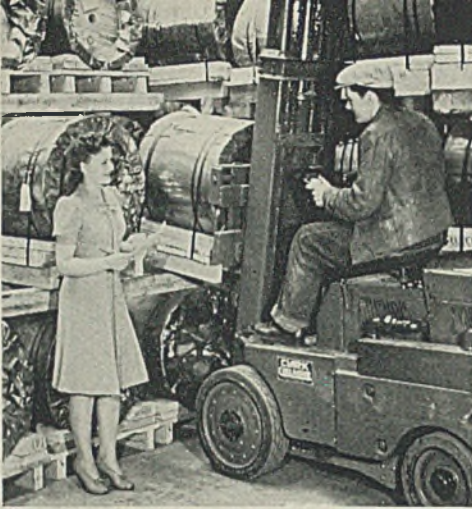
Speeding deliveries with unit packages and power handling equipment. Page 88.
