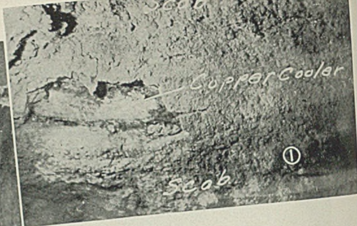
Fig. 1—Bronze bosh cooler protruding through scab. Water cooling of bosh is sufficient to maintain refractories
