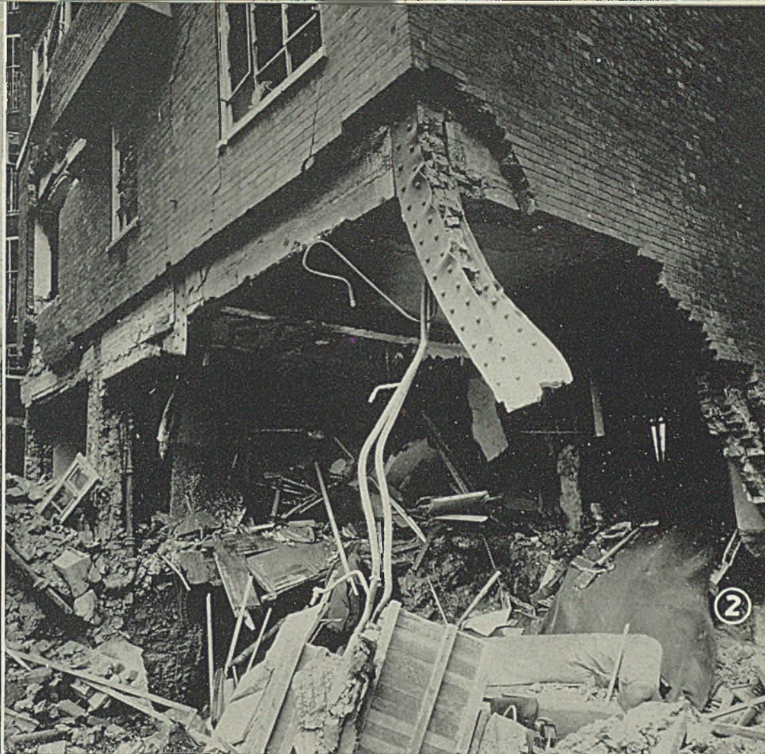
Fig. 1—These views show that steel-framed buildings have the ability to withstand severe punishment from bombing without damage to the structure as a whole. Crater indicates detonation occurred when bomb struck foundation walls in this apartment house at Westminster Gardens, S. W. 1.
