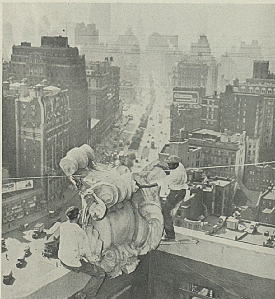
HIGH above Broadway and Seventy-third street in New York, workmen last week were removing one of the cornices which has adorned the Ansonia hotel for many years. Reason is to obtain the copper it contains for use in the war effort. NEA photo
