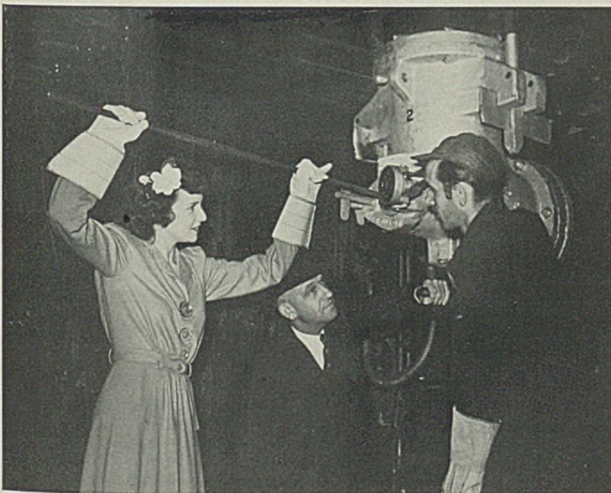
PITTSBURGH: Pretty Jean Rodgers aims a glowing hot rod into the tuyere and a U. S. Steel blast furnace returns to operation at Carnegie-Illinois Steel Corp.'s Clairton Works. The blowing-in ceremony came after rehabilitation of the giant furnace was achieved 21 days ahead of schedule. Miss Rodgers is a granddaughter of William Stewart, veteran blast furnace superintendent at Clairton. Others shown are H. W. Seyler, assistant general superintendent, center, and William Painter, hot blast man. U. S. Steel Corp. subsidiary photo
