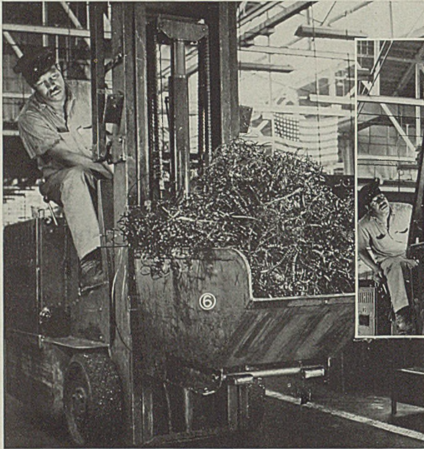
Fig. 6—Second step involves use of an industrial power truck which picks up the chip box and carries it to a nearby gondola carrying similar scrap. Metals are carefully segregated beginning at the machine tool. Scrap handling system salvages steel, aluminum, magnesium, brass and bronze
