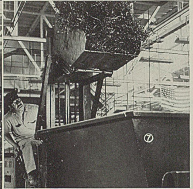
Fig. 6—Second step involves use of an industrial power truck which picks up the chip box and carries it to a nearby gondola carrying similar scrap. Metals are carefully segregated beginning at the machine tool. Scrap handling system salvages steel, aluminum, magnesium, brass and bronze
