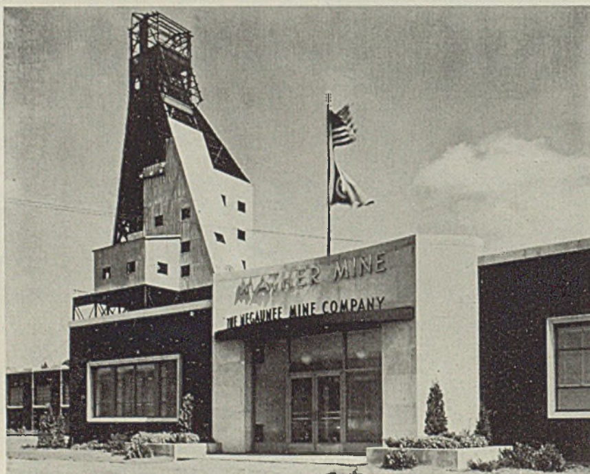
MATHER mine of the Negaunee Mine Co., Negaunee, Mich., has been provided a model $250,000 structure, designed and built by The Austin Co., to house surface facilities. A "change house," 60 x 280 feet, adjacent to the office building shown above, provides comforts for the miners. Head frame, in background, is 200 feet high above ground. Mine is owned jointly by Cleveland-Cliffs Iron Co. and Bethlehem Steel Corp.
