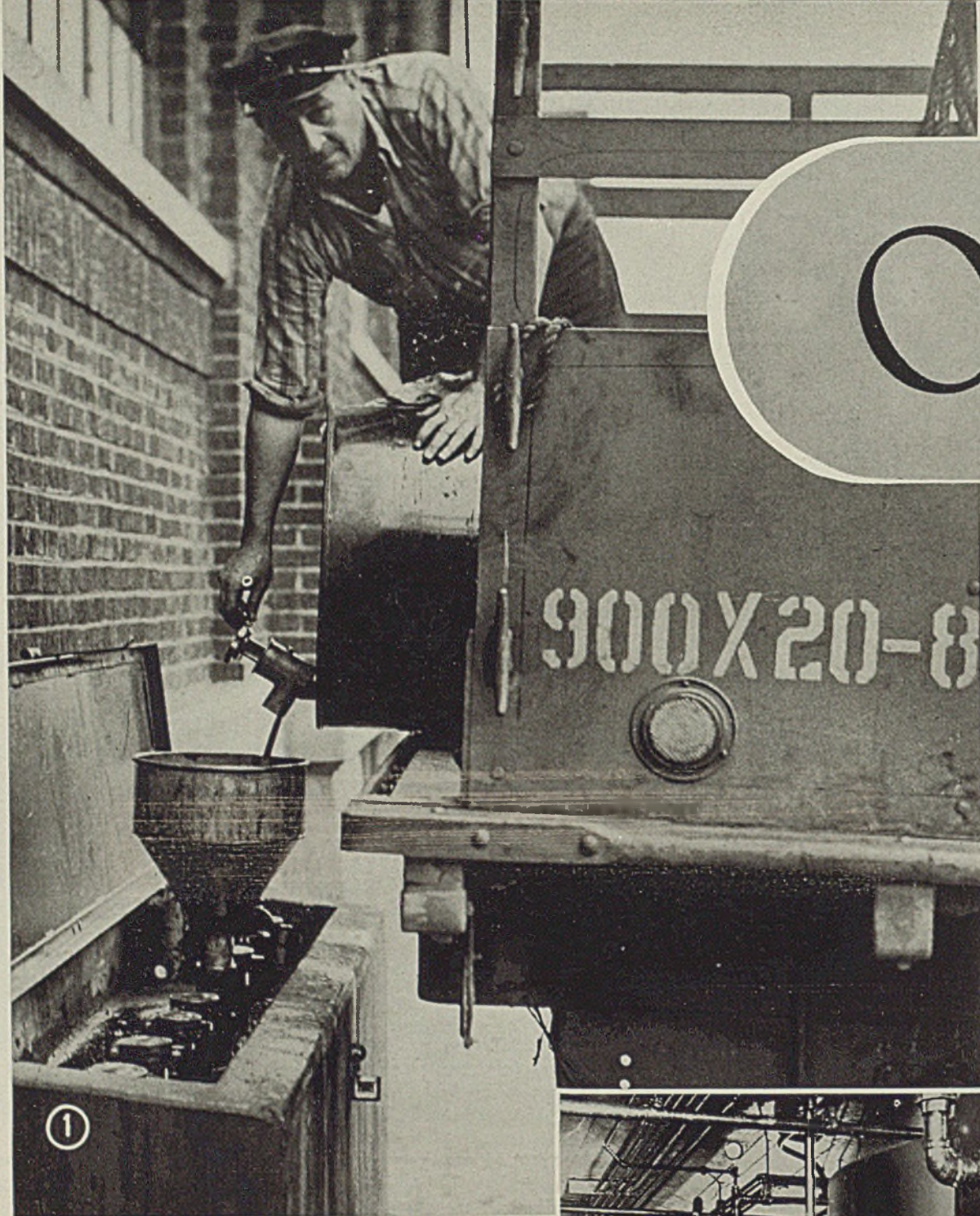
Fig. 1—The eight oil receiving lines are enclosed in this steel and concrete compartment for protection against fire, theft and other hazards
