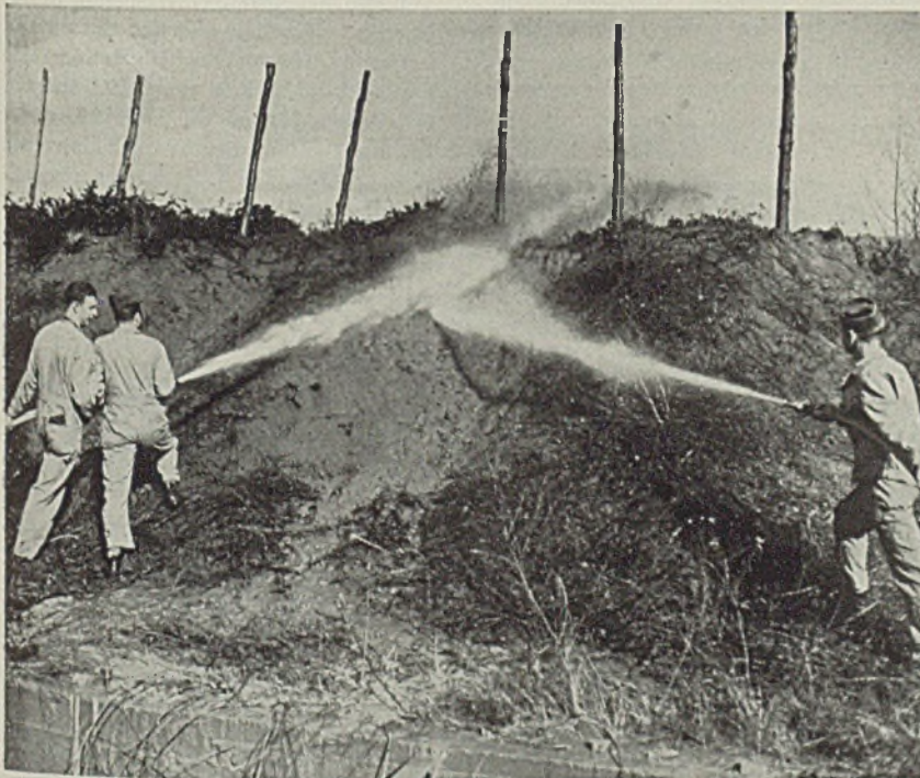
FIRING range butts at Fort Knox, Ky., "Home of the Armored Force," are now yielding precious metal deposits, in the form of bullets containing lead, copper, antimony, zinc and nickel, that have been fired by thousands of soldiers there in the past 20 years. One method of reclamation is by sluicing; in another, the ground is dug up, placed in a tumbler of water, bullets being screened out from mud. By this latter method salvage has averaged 100 pounds of metal per cubic yard. NEA photo
