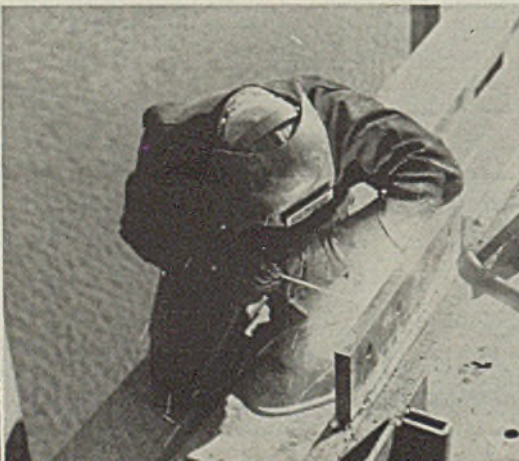
Hand welding is employed for much work, also, Union Melt machine being limited to application of downhand welds
