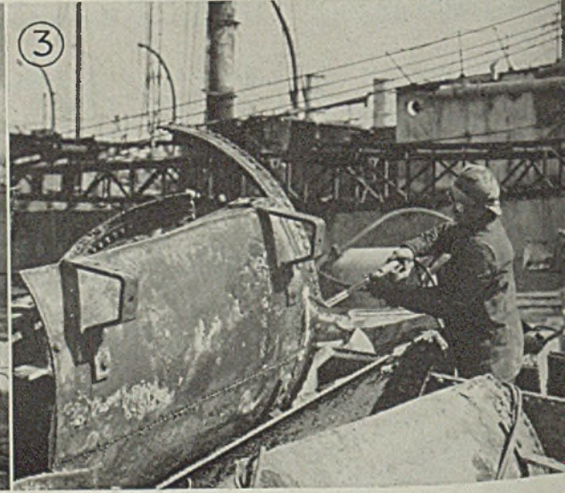
Fig. 4—To facilitate the scrapping operations, whole sections are cut free and removed for further cutting away from the ship
