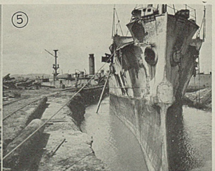
Fig. 5—End view of old battleship in process of being cut up for scrap. Note railroad running alongside for fast transportation of scrap by means of locomotive cranes and cars.
