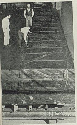
Laying out patterns on large section of plate for prefabrication of tank lighter component. Photo by Higgins Industries, Inc.
