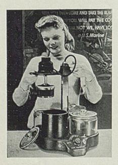
cleaner is agitated by a powerful, aircooled fractional horsepower motor. Its work basket is 2¼ inches in diameter by 5% inches inside diameter.
