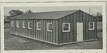
TASK FORCE BUILDING: Specially engineered by the Tennessee Coal, Iron & Railroad Co. in co-operation with Army and Navy personnel for use by our armed services overseas steel utility structures such as shown in the accompanying illustrations are designed so that component parts nest together and require a minimum of shipping space. A 20 x 50-foot unit requires slightly less than  $5\frac{1}{2}$  tons of steel and all parts take only 225 cubic feet of shipping space.
