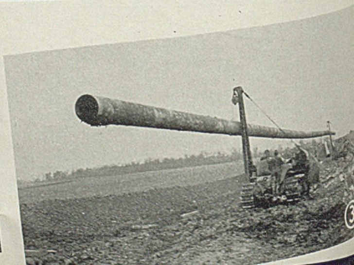
Fig. 3—Two tractors are shown carrying a 150-foot section to the end of the main line for tying-in
