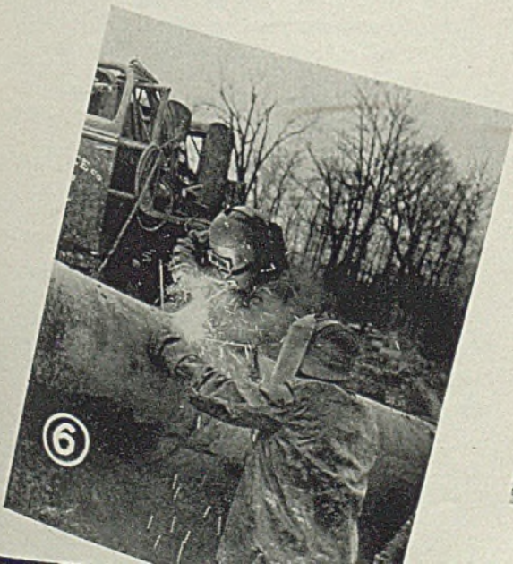
Fig. 6—Two operators make final roll welds joining a new section to the main line
