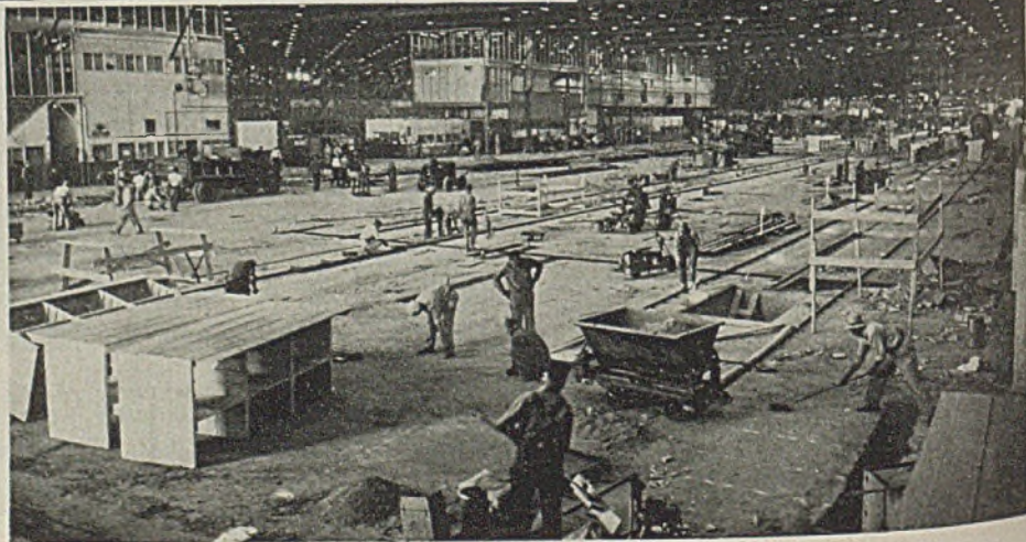
Final assembly hangar at Lockheed plant, right, was completely stripped before installation of conveyors. Eight days later the installation was completed, photo showing the plant midway in the job. In the interval, assembly operations were moved outdoors
