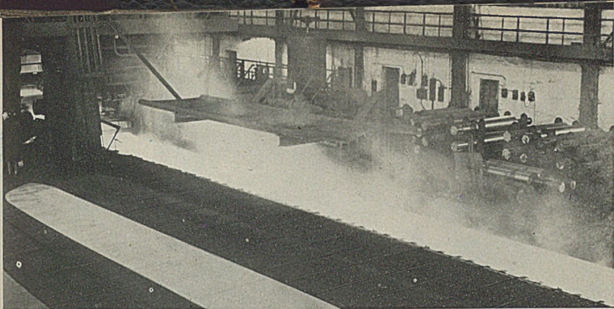
Finished floor plate from continuous mill being laid down on cooling bed
