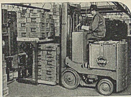
Tiering on racks allows access to underneath pallet load with Baker Fork Truck.
