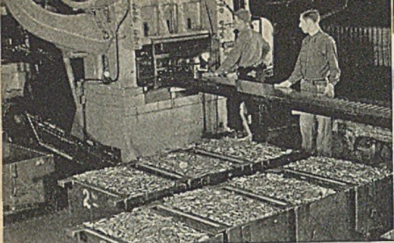
The press stamps landing mat sections out of heavy gage Inland sheets. The much-needed scrap goes back to the steel mills.
