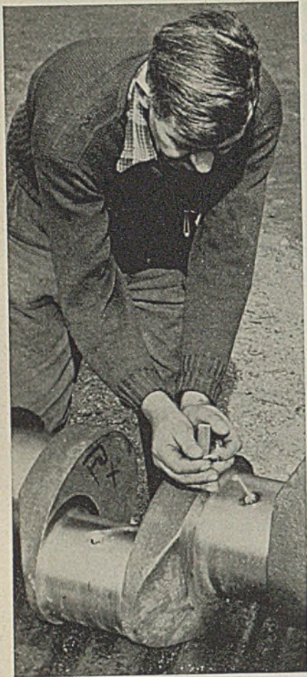
Fig. 1 (Above)—Dynamiter ignites fuse after tamping dynamite into oil hole and inserting cap. Less than thimblefull of dynamite is needed
