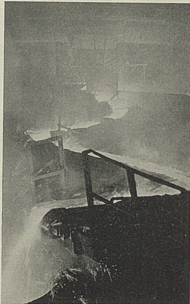
Fig. 1—Familiar scene at blast furnace at casting time
