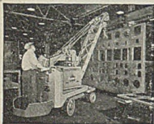
In erection of control panels, Baker releases overhead cranes for other work.
