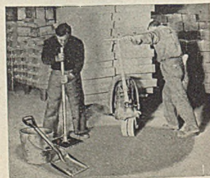
Floor patch takes traffic immediately
