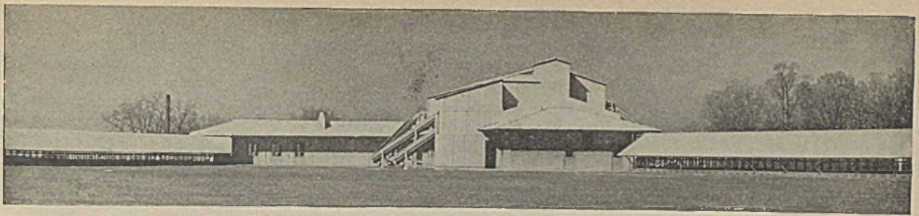
A typical bag loading house with one covered walk leading to the canteen and the other to the storage magazine. Note chutes for quick exit from second story
