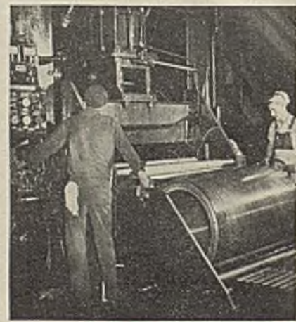
The rolling mill produces aluminum sheets, rods and shapes for aviation
