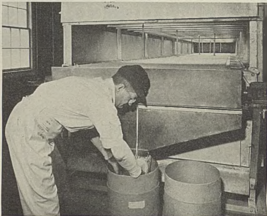
"Dry" end of infra red ray ball powder dryer at plant of Western Cartridge Co.
