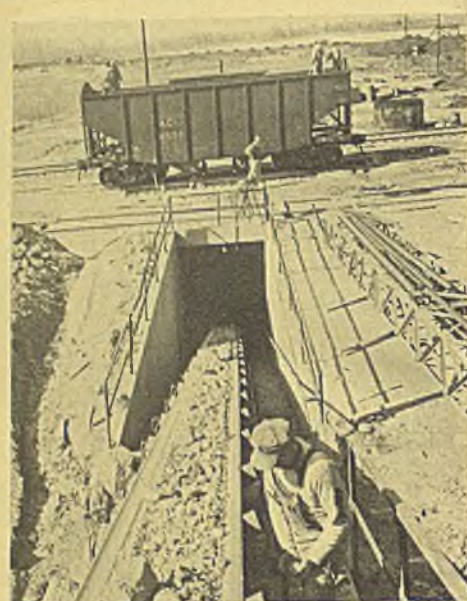
1 Bauxite and all other raw materials are received at the plant by railroad
