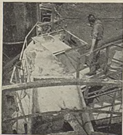
At the left liquor from precipitation tanks flows into hydroseparators. At right are two "white mud" thickeners. Building beyond is for washing and dewatering
