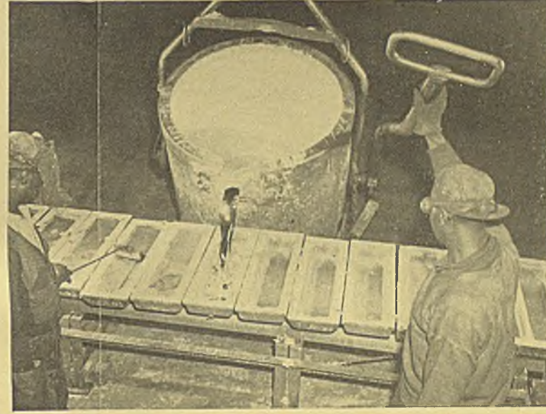
11 Crucibles are brick-lined and hold 3,000 lb. Molten metal is cast into 52 lb. pigs and transferred by truck to the yard outside
