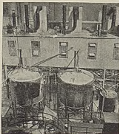
At the left liquor from precipitation tanks flows into hydroseparators. At right are two "white mud" thickeners. Building beyond is for washing and dewatering
