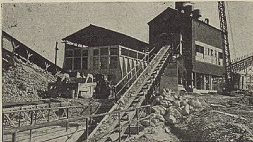
Ore is handled and stored by an elaborate system of conveyors. It is screened and the oversize crushed in building on the right. Bedding building is at left
