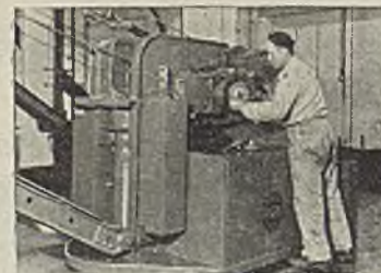
Removing the rotor disc from the magnetic disc brake for monthly inspection.
