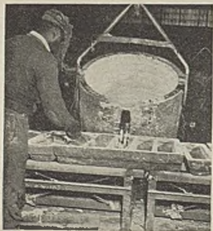
Molten aluminum is cast into 52 lb. pigs and moved to adjacent rolling mill
