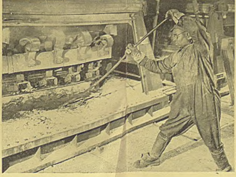
10 Rectangular Soderberg continuous electrodes are used in the cells. Cells are tapped for molten metal every third day
