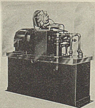
Electric-hydraulic filter closer
