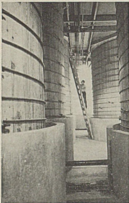
Buna S latex is bulked and blended in these huge wooden tanks
