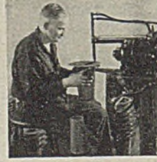
Welding Pipe Line Strainers
