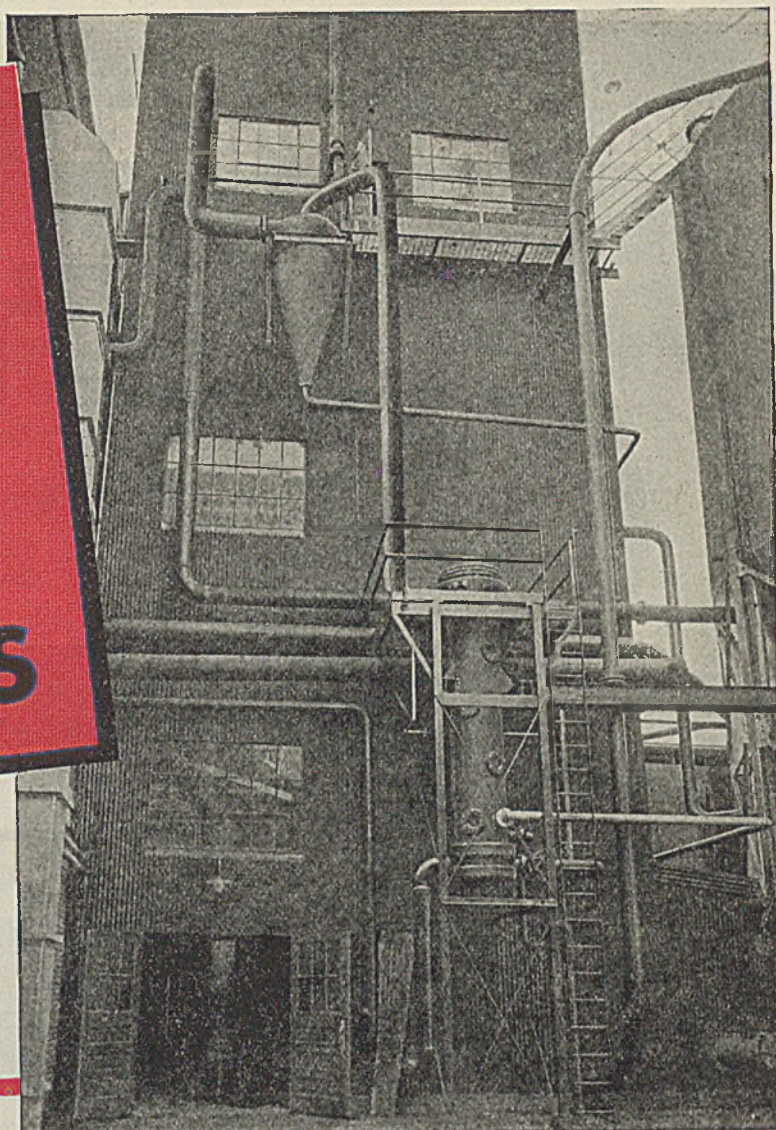
This unit, in operation at a large Southern pulp mill, is designed to recover 600 gals. of crude turpentine per day.
