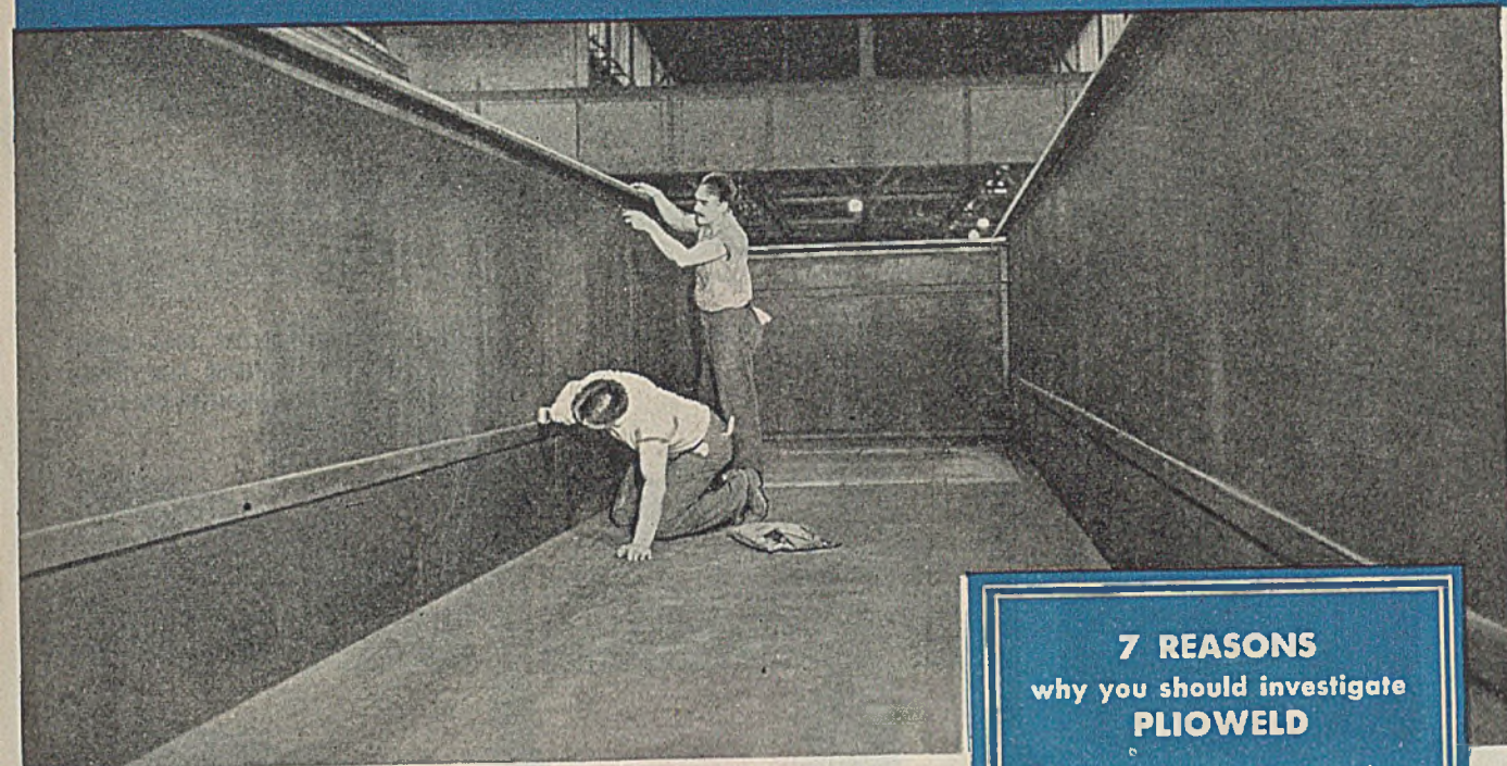
Goodyear experts applying Plioweld lining to large pickling tank.
