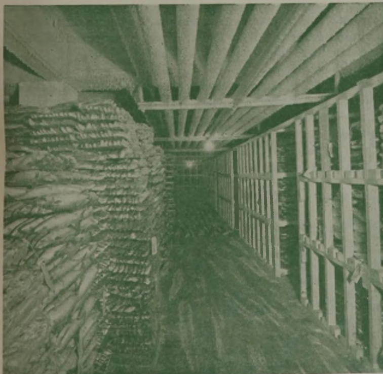
Courtesy, Commonwealth Ice and Cold Storage Company Storage for Frozen Fish, Showing a Section of Bins Used for Small Lots
