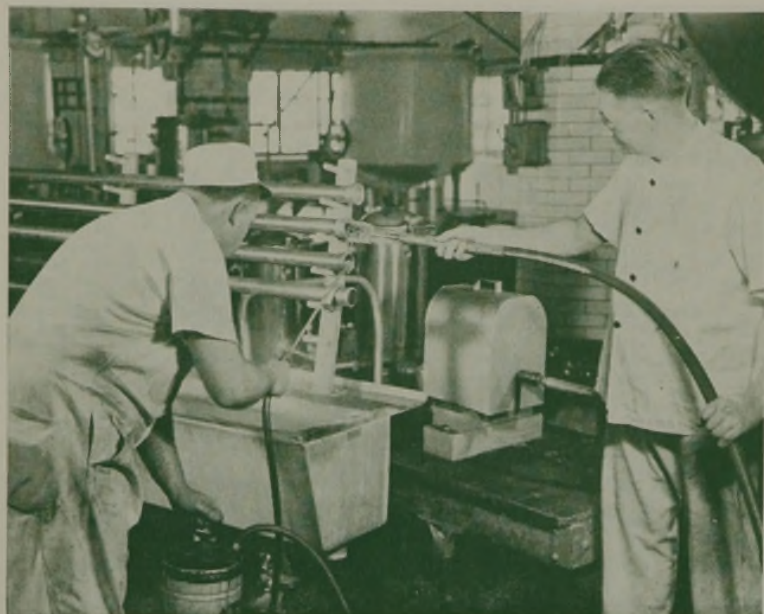
Spraying Sanitary Pipes with Acid Cleaner Solution, Subsequently Cleaned with Motor-Driven Bristle Brush
