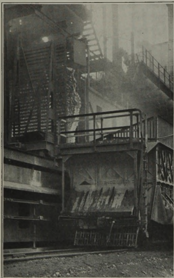
Coke Being Pushed from a By-Product Oven into a Hot Car
