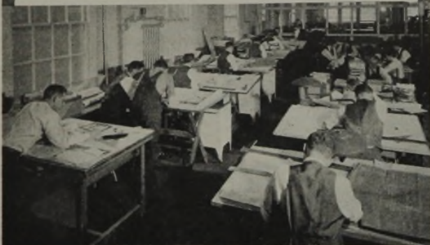
One of the engineering rooms at S. Blickman, Inc.
