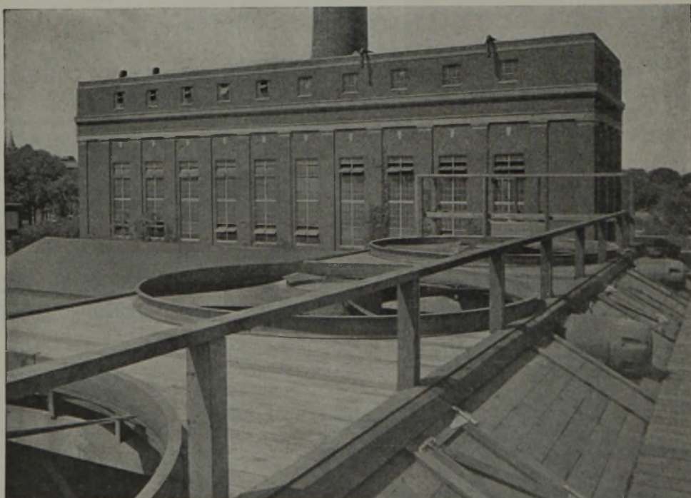
View of Induced Draft Fans Showing Fan Mounting and Top Deck Construction.
