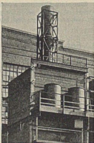
47' high all-carbon electrostatic precipitator
