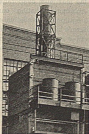
47' high all-carbon electrostatic precipitator
