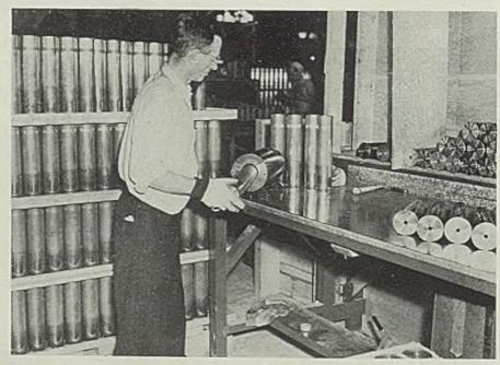
Three-inch shells are measured by an employe in a Los Angeles stamping plant, a part of which has been turned over for the manufacture of defense materials. Acme photo
