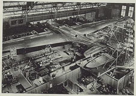
■ Nearly completed in Douglas Aircraft Co.'s Santa Monica. Calif., plant is the army's B-19 super bomber, claimed to be the largest airplane in the world. Capable of taking off with a gross weight of 164,000 pounds, the ship soon will undergo army tests. It is powered by four 2000-horsepower Wright Duplex Cyclone engines and can carry enough gasoline for a 7500-mile nonstop flight. Its armament is a closely guarded government secret
