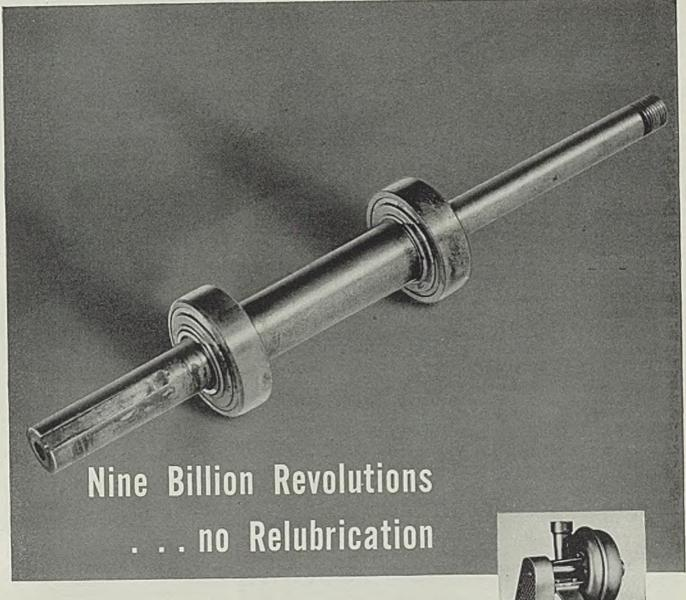
WHEN they mounted these New Departure Self-Sealed ball bearings on their blower shaft for testing, the Allen-Billmyre Company of South Norwalk, Conn., were looking for bearings that would give them dependable, long-life operation minus the cost and bother of frequent lubrication.
