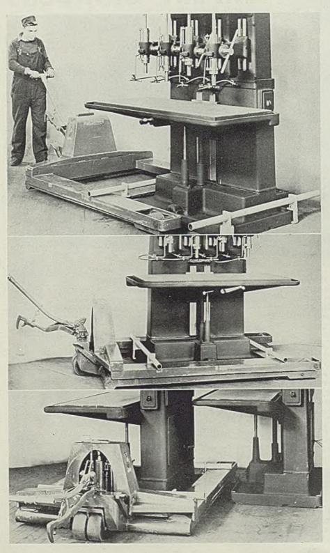
side one already in position. Clearances are small. No crane or lift platforms are used. The method provides a neat compact arrangement in space that formerly would not be available for storage. All storage aims at leaving a minimum of unoccupied space, and Fig. 4 illustrates how close the machines can be placed by this method. Even with minimum clearances, there is slight possibility of damage to machines already in place or to the machine being stored.
