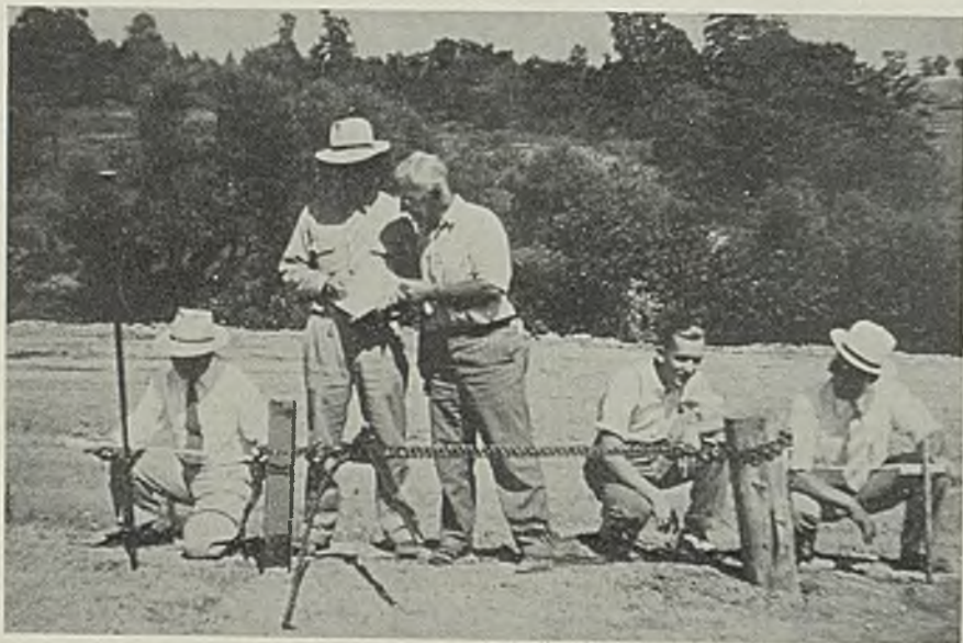
■ Before steel posts were installed for guard rail supports on the new Harrisburg-Pittsburgh turnpike, the tug-of-war, shown above, was staged between wood and steel posts. At the first test, the steel post had tipped only \frac{3}{8} -inch while the wood post had moved 2\frac{1}{2} inches. When the tip of the steel post had increased to 2\frac{3}{4} inches, the wood post had yielded entirely. Steel post was driven while the wood post was set in well-tamped earth. Steel post employed was a standard Bethlehem 7\frac{1}{4} -pound section
