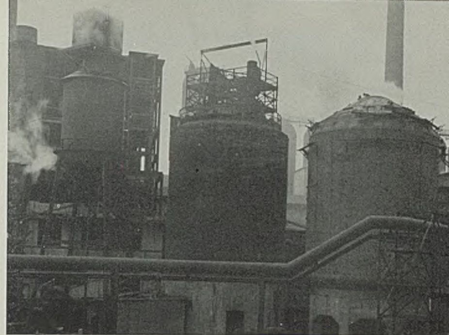
East elevation of high-pressure boiler plant extension. The duplicate Cochrane 160,000-gallon per hour softener is shown at right
