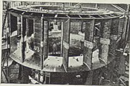
Weld fabricated sub-assemblies of ribs and bracing structure.
