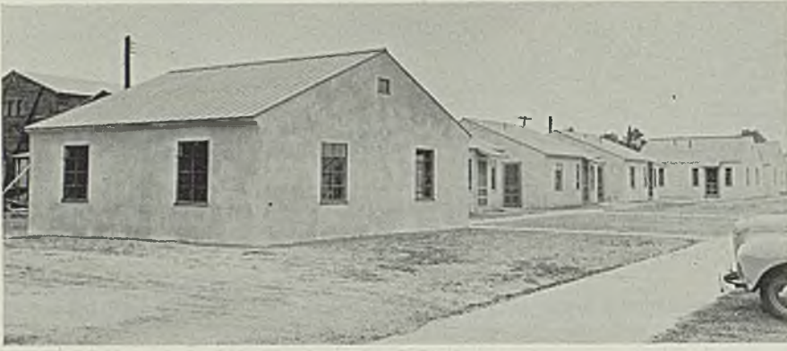
■ Fifty of these five-room homes were built for the navy department at Norfolk. Frame is steel. Exteriors are Gunitite sprayed over Firtex panels
