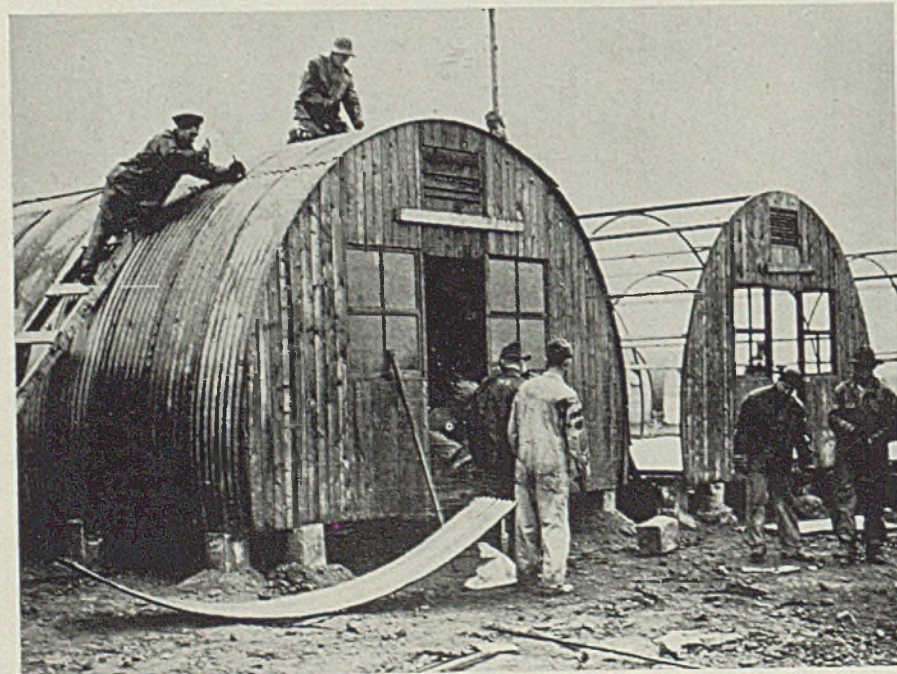
American marines and British soldiers working together building huts of galvanized steel and wood in preparation for the winter in Iceland. Photo passed by British censor
