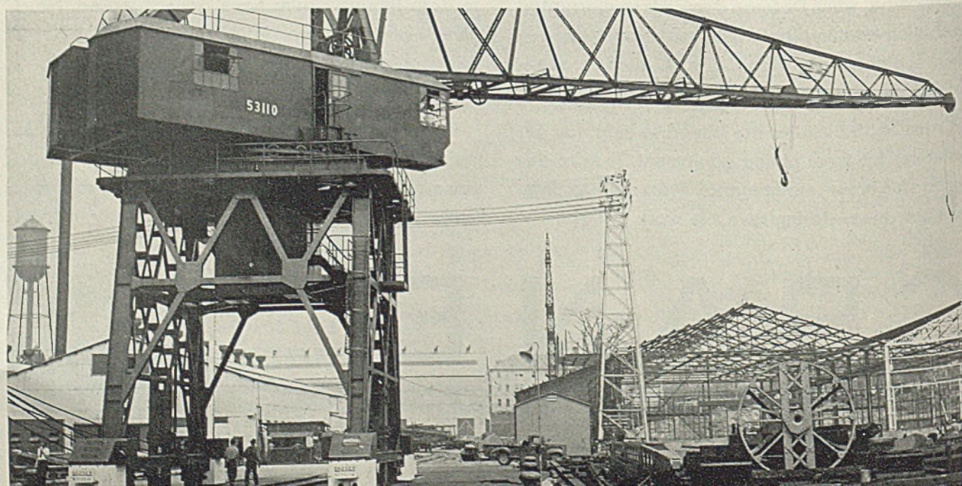
Fig. 3—All-welded screw luffing crane built with rail clamps
