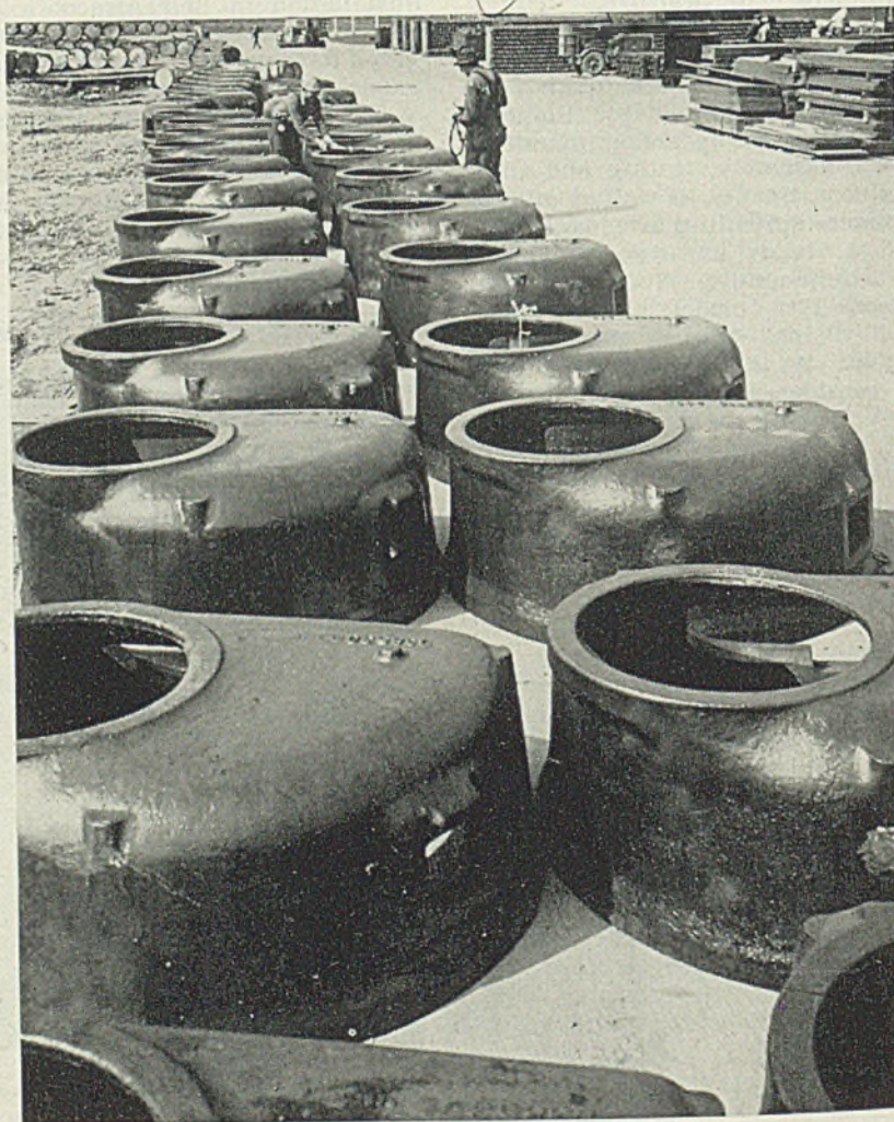
■ Ready for installation in 28-ton Chrysler M-3 tanks, these 4000-pound turret castings have just been received at the huge Chrysler tank arsenal in Detroit. More than 10,000 men are engaged at this plant in production of the medium "rolling arsenals." OEM photo
