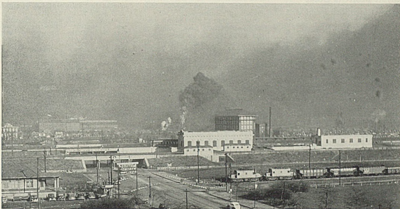
■ GARY BLACKOUT: Ordinarily Carnegie-Illinois Steel Co.'s Gary, Ind., works, in the background, are clearly visible from the point at which this photo was taken. Company in co-operation with the Army has conducted "daytime blackout" smoke screen tests to see how effectively the plant could be concealed from enemy bombers. The smoke screen is developed by tar and wet coal in the furnaces, with switch engines also used as smudge pots. Tests were reported successful. Railroad bridges and depot in the foreground were not screened. NEA photo
