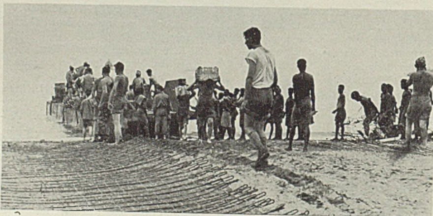
STEEL matting is laid on the beach at Guadalcanal Island to prevent heavy vehicles from sinking into sand as they are landing from vessels. This picture shows natives helping the United States Marines. U. S. Marine Corps photo
