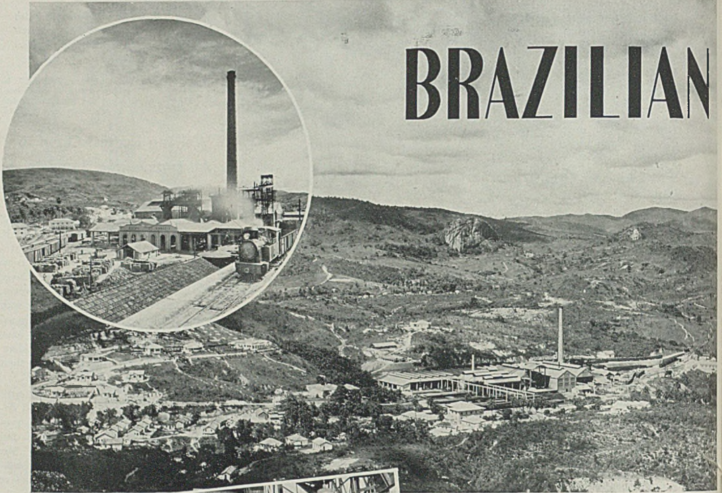
Top left—Three hand-filled charcoal furnaces supply pig iron for cupolas serving the centrifugal pipe machines
