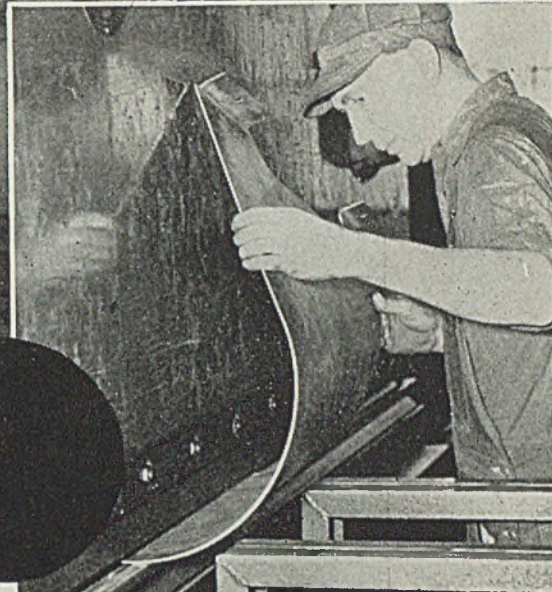
Forming an exhaust housing with curvature of 8-inch radius.
