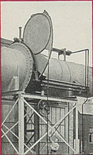
One of four 120" Three Tube Thermal Valves
