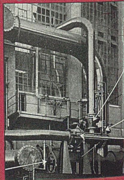
Thermal Valves in Vertical and Horizontal Gas Mains
