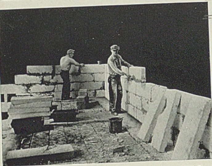
INSULATION FOR TEMPERATURES TO 1900° F. J-M Superex Blocks have long been standard for this service. High heat resistance, low thermal conductivity. Sizes 3" x 18", 6" x 36" and 12" x 36"; from 1" to 4" thick.
