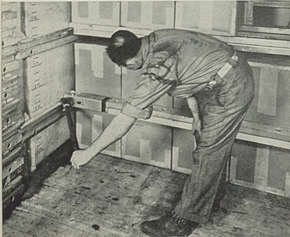
Fig. 4—This tool engaging the teeth in the rack permits tightening load securely to prevent loads from becoming loose and hammering upon themselves. Thus the loader prevents the cause of most shipping damages
