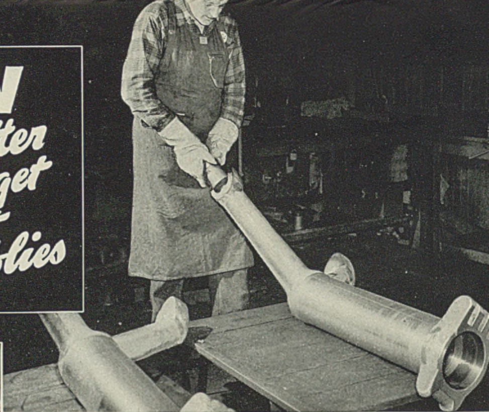
(Above) Operator merely slips chilled plug into heated strut for a permanent shrink-fit assembly.
