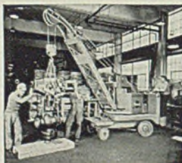
Baker Crane Truck spotting a large valve in position for crating.
