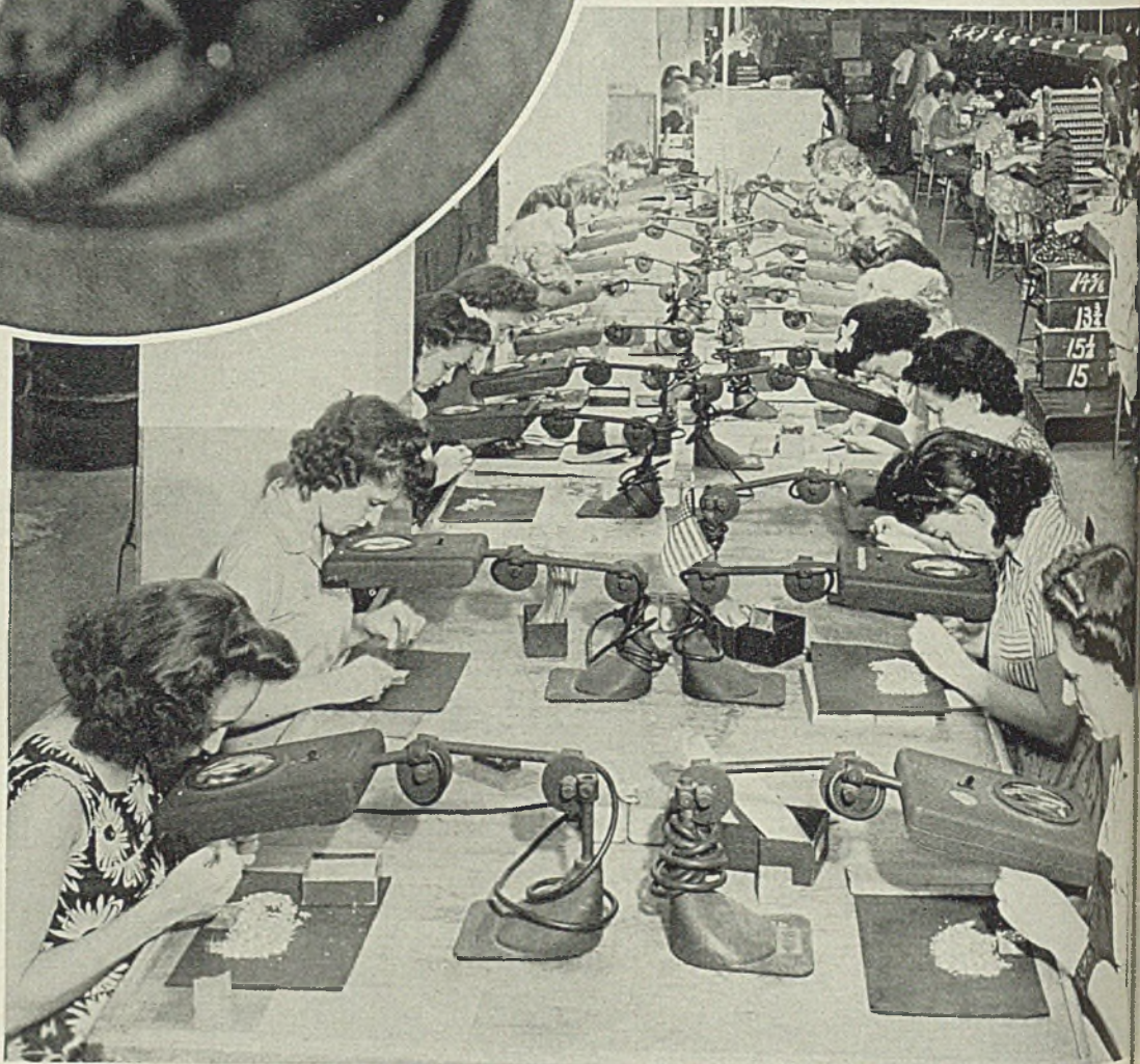
Above—Closeup of what inspector sees through magnifier which permits detection of flaws invisible to the unaided eye
