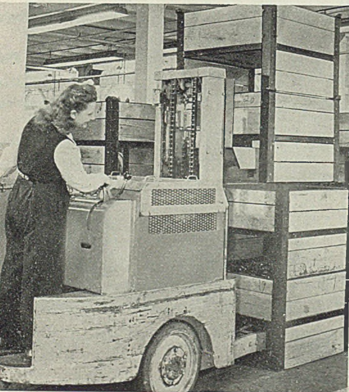
Left below—Accurate teamwork of hands, eyes and feet is necessary in tiering but the women operators quickly become experts Right—Skid boxes are the usual handling unit through processing
